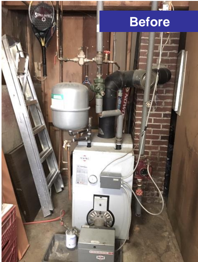
Oil boiler with coil
