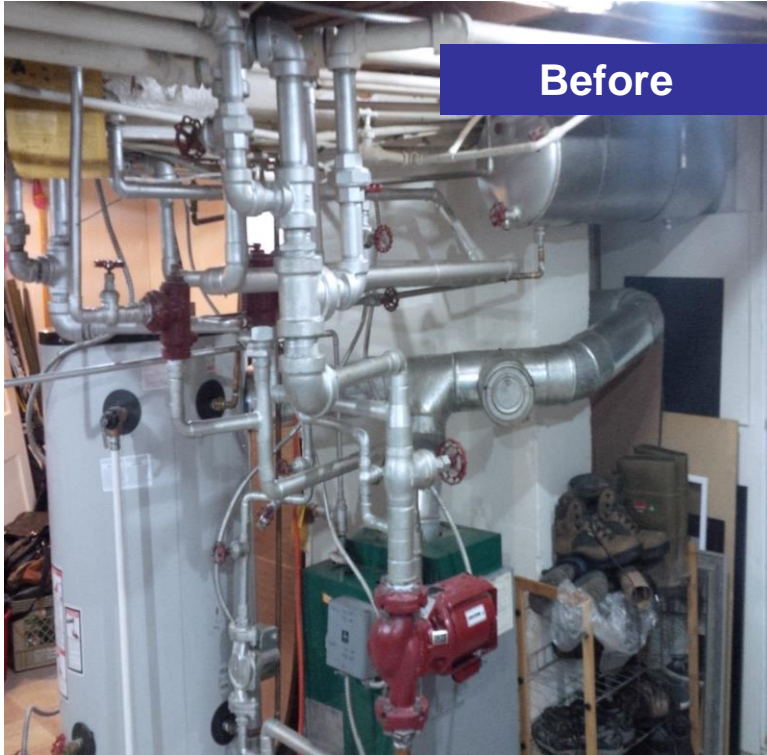
Oil boiler with electric water heater
