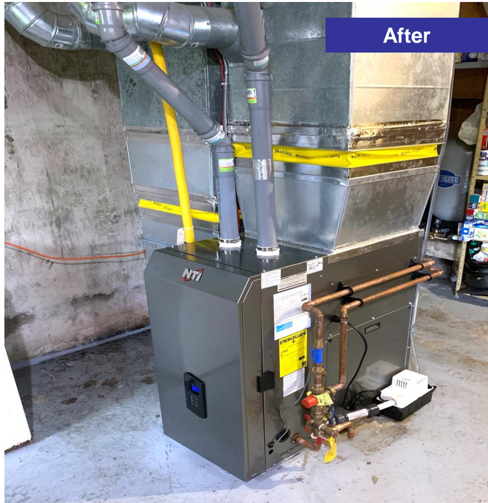
Propane furnace with tankless water heater
