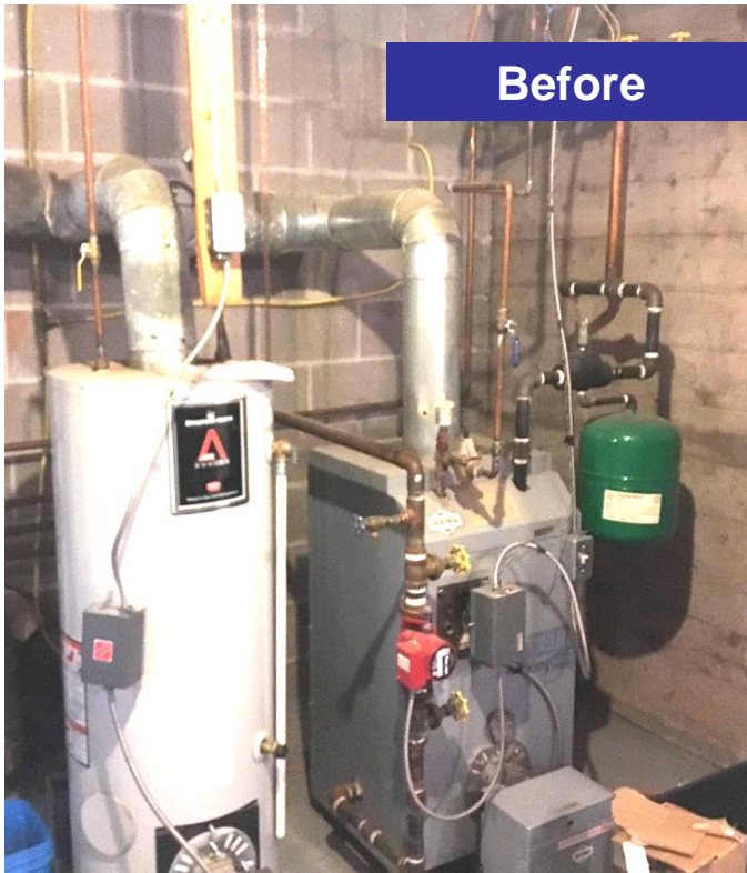
Oil boiler with oil water heater
