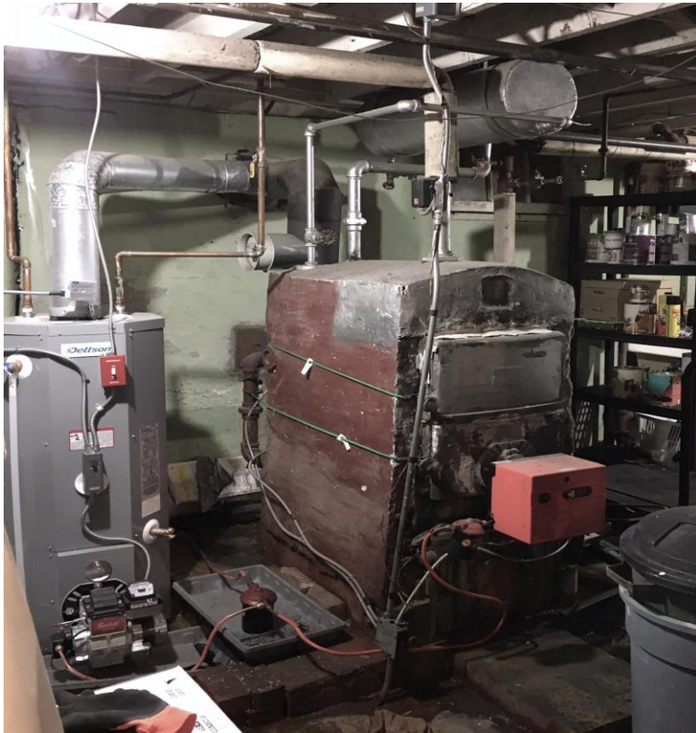
Oil boiler with oil water heater
