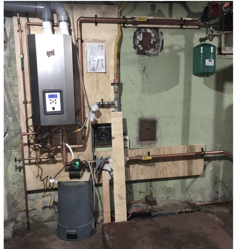
Propane boiler with tankless water heater built in
