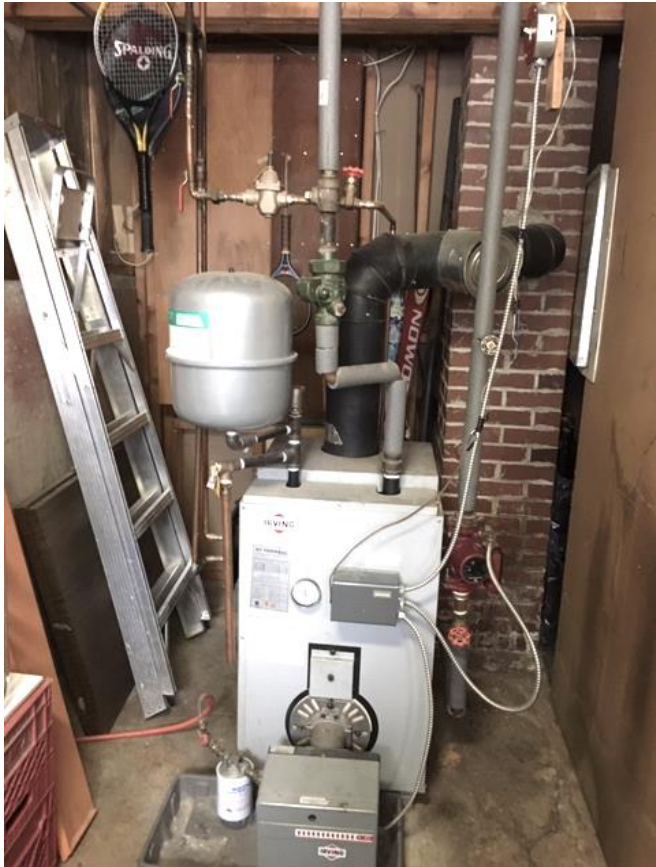
Oil boiler with coil
