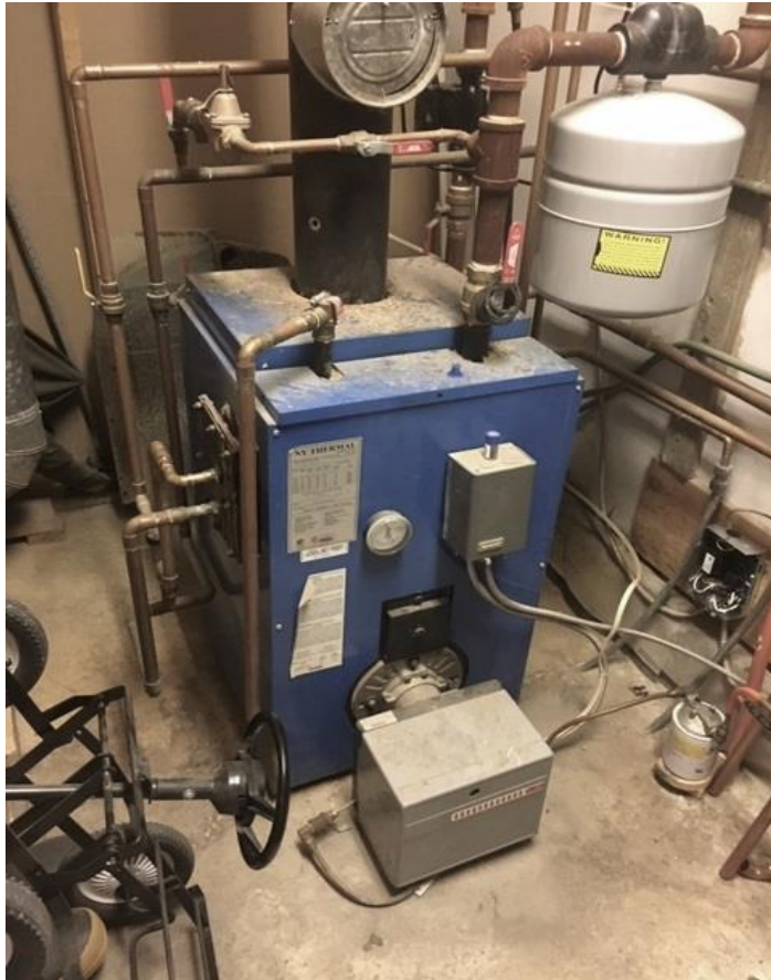
Oil boiler with coil
