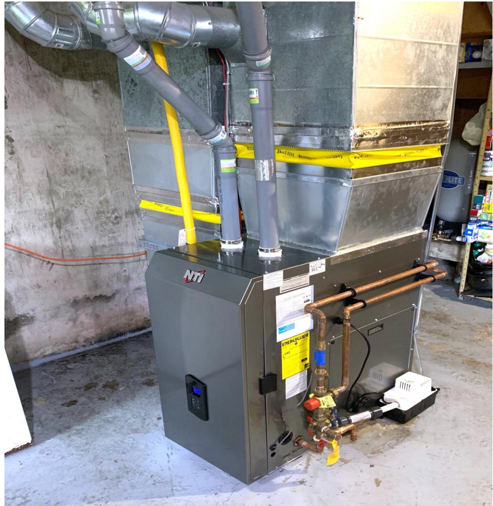
Propane furnace with tankless water heater
