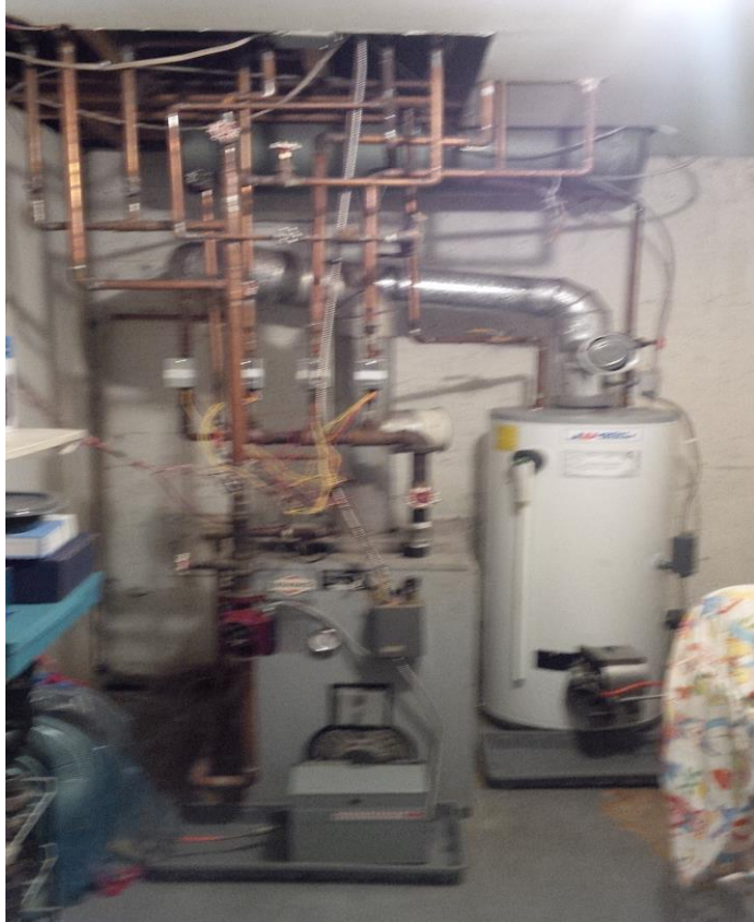
Oil boiler with oil water heater
