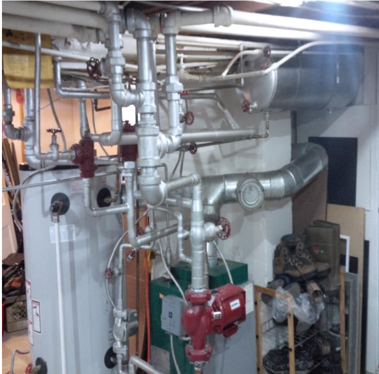
Oil boiler with electric water heater
